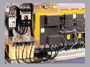
Power cabinet is totally enclosed and isolated from from plant atmosphere, reducing the amount of airborne contaminants that can settle on drives and electrical components.This increases the life of electrical components and helps avoid power failures. Base mounted fans pull air in through the cabinet, cooling heat sinks so drives can be enclosed safely.
