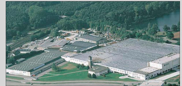
Main facility in Malterdingen
