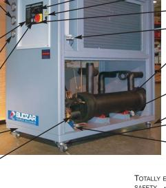
MOTOR CIRCUIT PROTECTORS (NOT JUST FUSES) PROTECT PUMP MOTOR AND COMPRESSOR ELIMINATES NUISANCE FUSE FAILURE AND FANS
